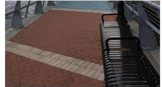
Per the South Bank paving precedent, a double row of brick pavers at 4" x 8" x 2-3/8", offset by approximately 1/2", shall be used when different paving patterns meet or when an interpretive paving area meets an existing or new paving pattern.
