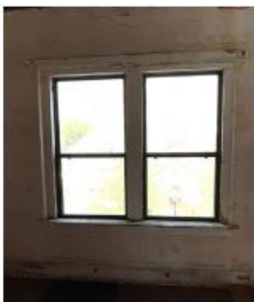
Front wall window with trim and plaster
