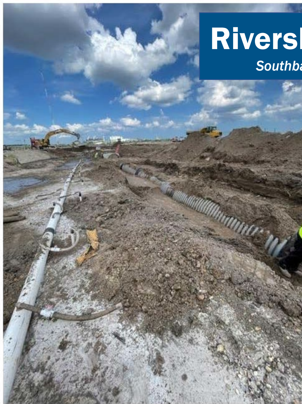
Installing 48" storm drain on Broadcast Place from ST-37 to ST-35.
