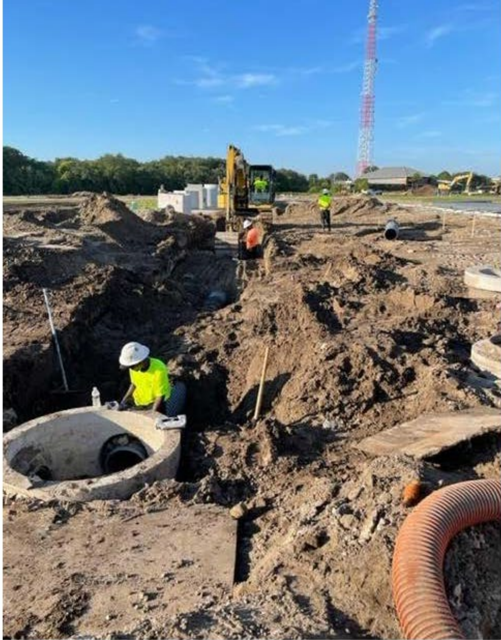
Installing 15" storm drain and installing structure ST-51 on Health Walk Way.
