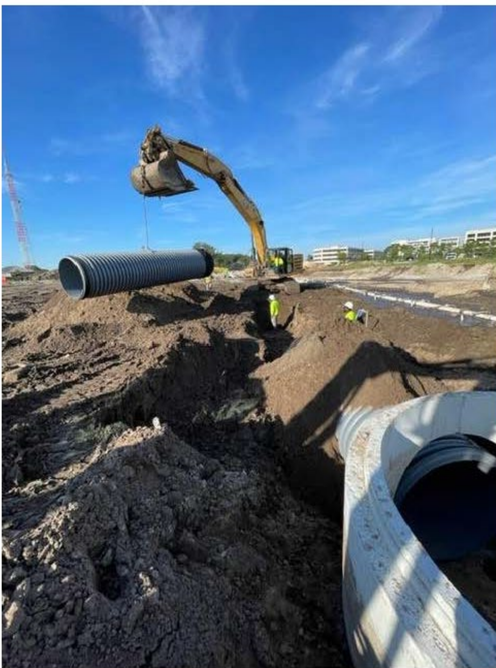
Installing 48" storm drain on Broadcast Place from ST-37 to ST-35.
