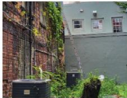
Partial view photo of rear elevation
