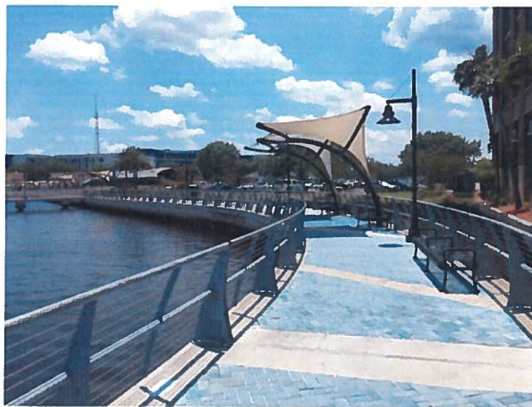
Existing Southbank Riverwalk railing and materials.
