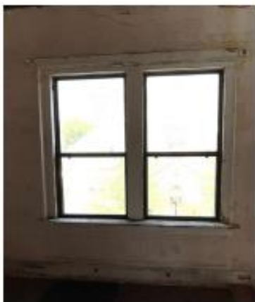
Front wall window with trim and plaster
