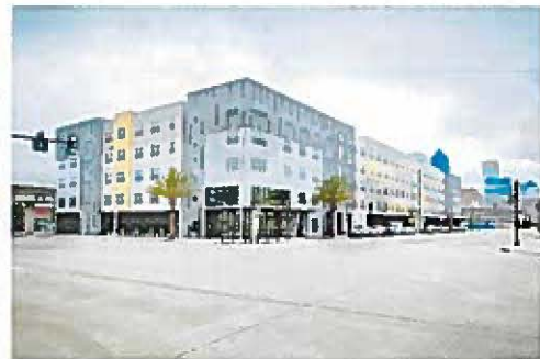
Lofts at LaVilla
