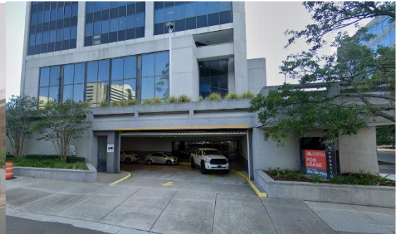
Bay Street Side
