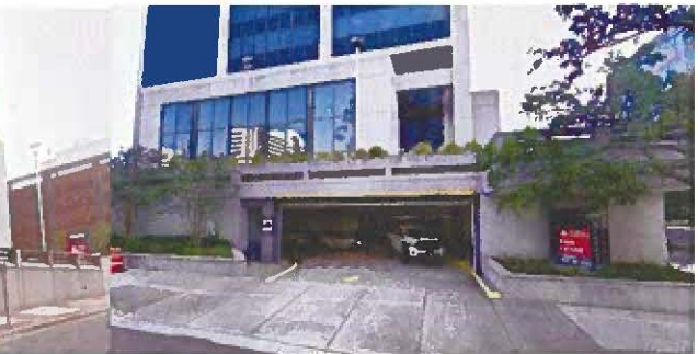
Bay Street Side
