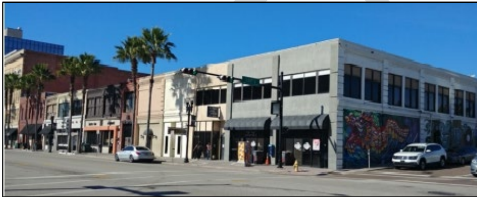
Figure 1. 333 East Bay Street
