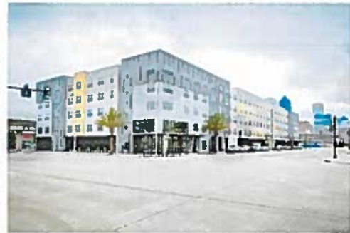
Lofts at LaVilla
