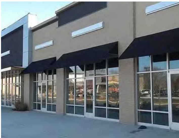
Do Not - Opaque, translucent and highly tinted windows do not contribute to the vitality of the sidewalk.
