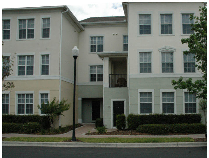
Do Not - Ground level units are missing the additional privacy or setback created by raised footprint.
