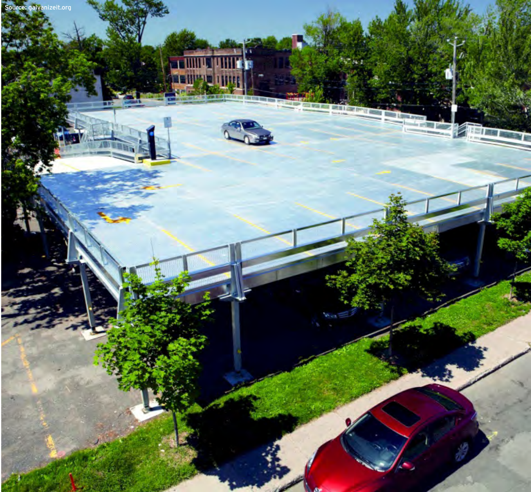
Single-level parking structure built over existing surface parking lot.
