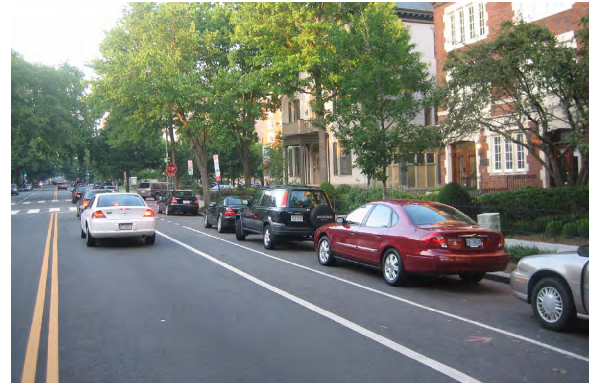
Bike lane added between travel lane and on-street parking
